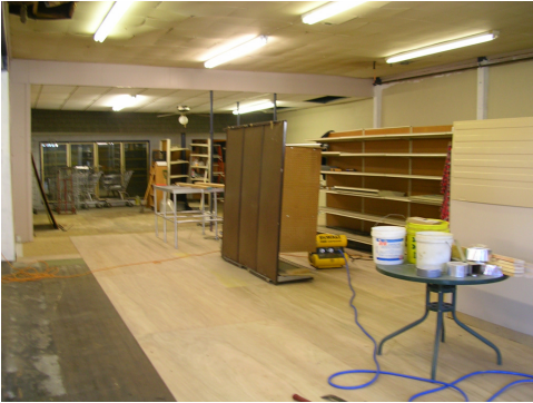
Renovations at Cullom Community Market.
